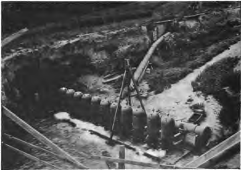
FIG. 18.—Battery of Hydraulic Rams, Yakima Valley, Washington.
